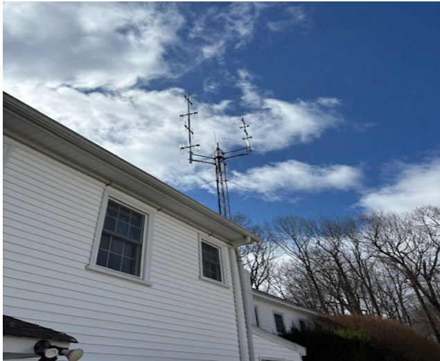
New Local Antenna for All Channels of Town Office
